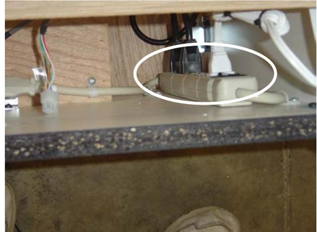
**Figure 2** Circuit Breaker Power Strip
